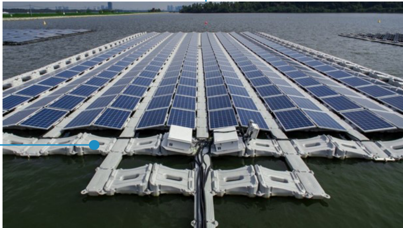
Floating solar panels installation
