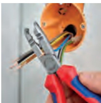
Cutting when shortening single conductors
